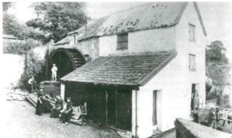
Raleigh Mill, Pilton. The launder that served this overshot wheel ran along the top of the wall to the left of the waterwheel.
