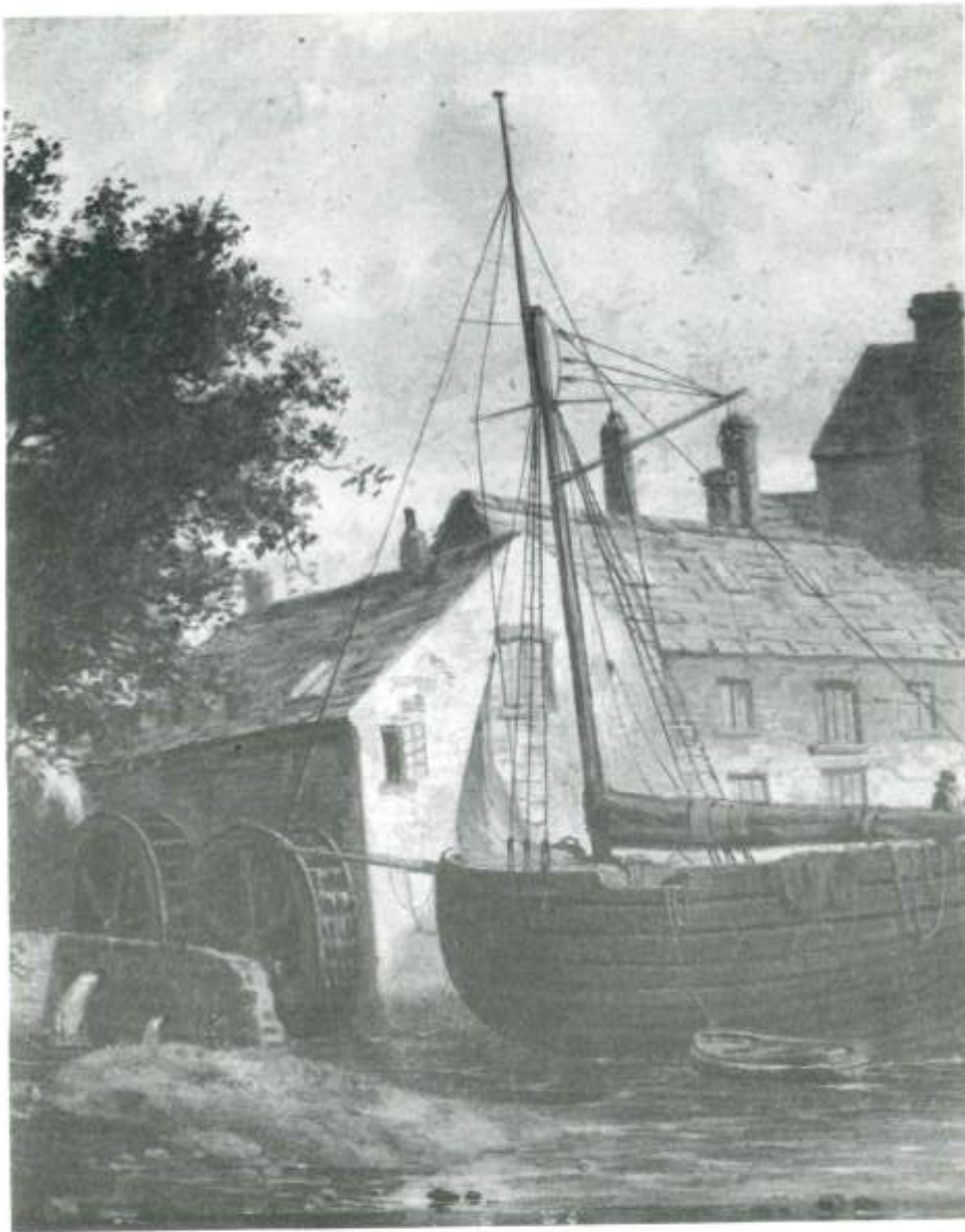
Town Mills (also known as Port Mill), Barnstaple, painted by Joseph Kennedy, probably between 1880 and 1885 when the building was pulled down. It was the predecessor of the Victorian Watermill on Baker's Quay, and probably was on a slightly different site. Note the two waterwheels in tandem. (Reproduced by permission of Mr. J. Lomas).
